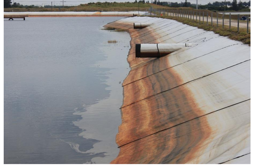
South Bottom Ash Pond (south side, looking east)
