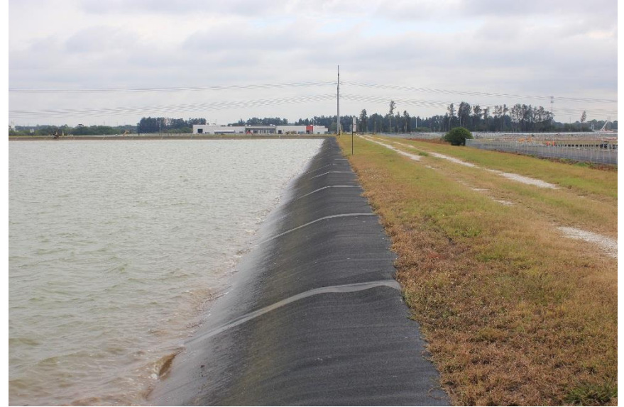
Long Term Fly Ash Pond (south side, looking east)
