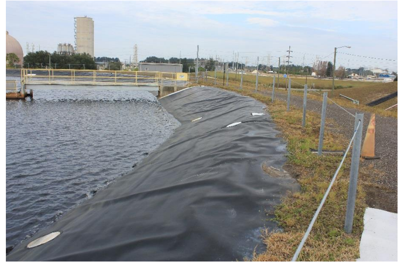
Bottom Ash Suction Pond (east side, looking north)
