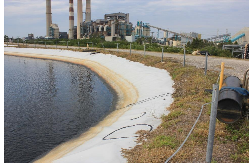
North Bottom Ash Pond (north side, looking west )
