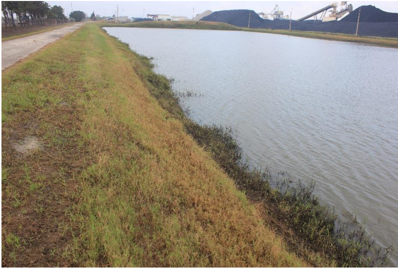
East Stormwater Pond (south side, looking west)
