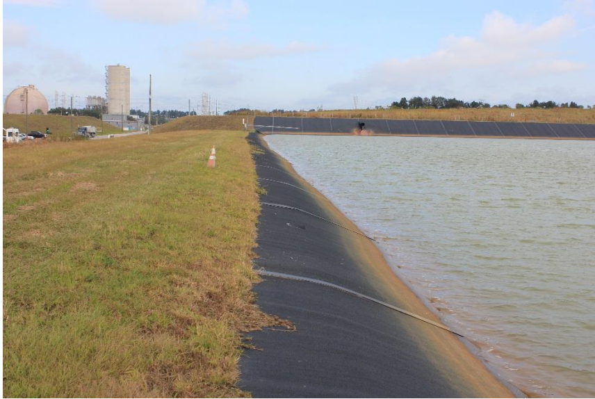
Long Term Fly Ash Pond (west side, looking north)
