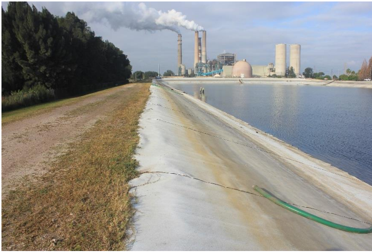
South Recycle Pond (south side, looking west)
