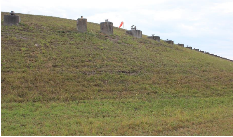
North Bottom Ash Pond (west side, looking east)
