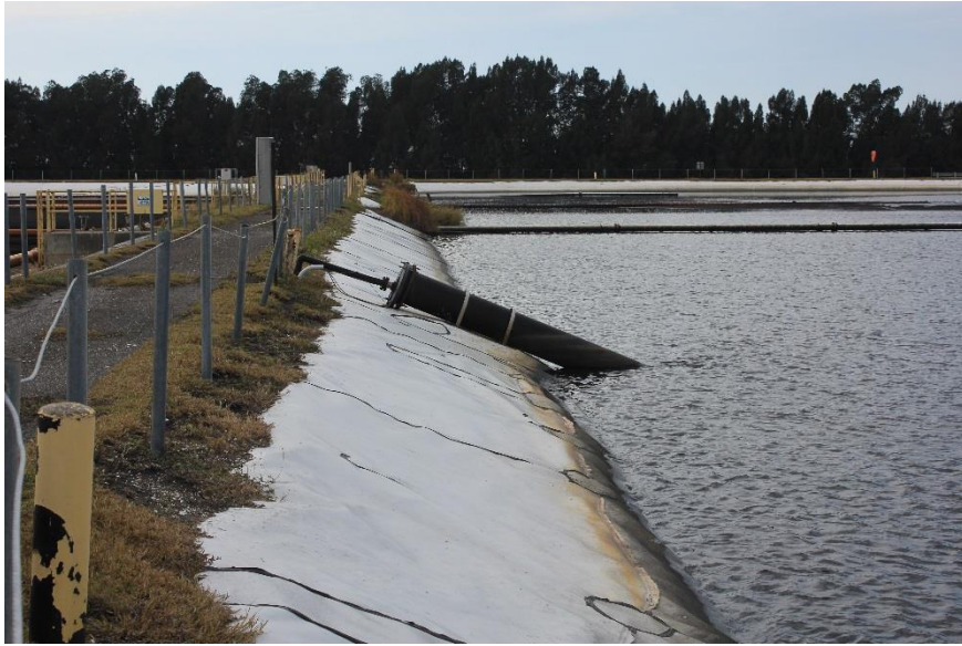
North Bottom Ash Pond (south slope, looking west)
