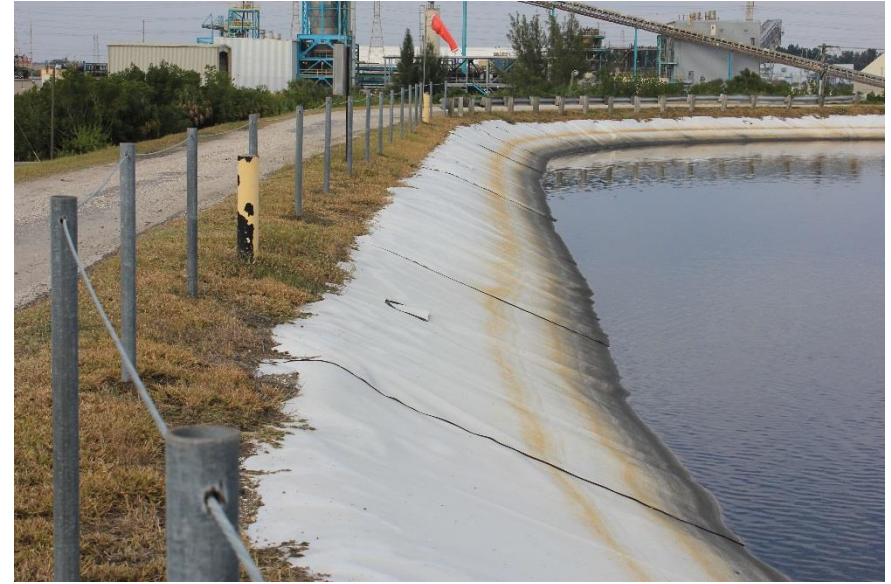
North Bottom Ash Pond (west slope, looking north)
