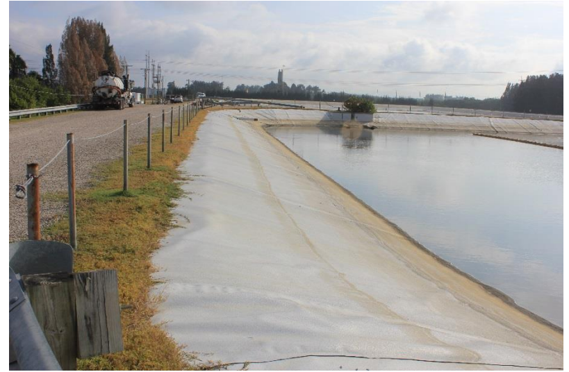
Recycle Settling Pond (north side, looking east)
