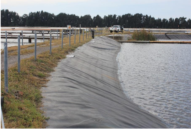
Bottom Ash Suction Pond (south side, looking west)
